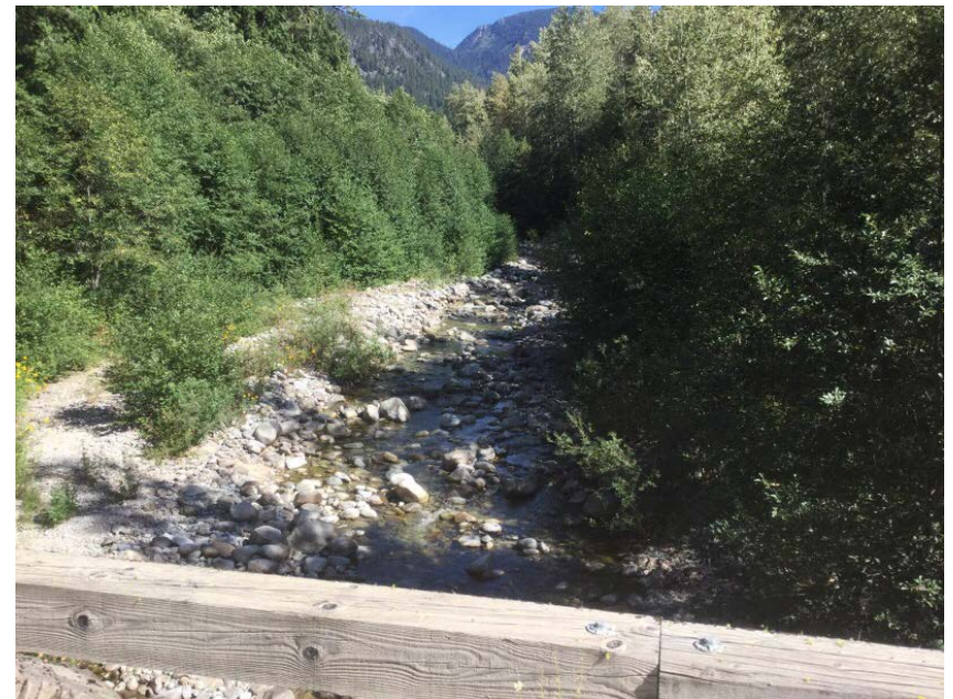
Looking upstream from deck
