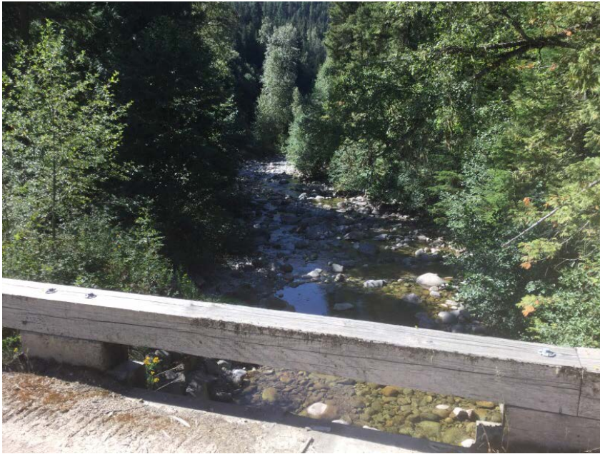
Looking downstream from deck
