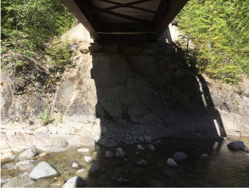
Right Bank Abutment when facing downstream
