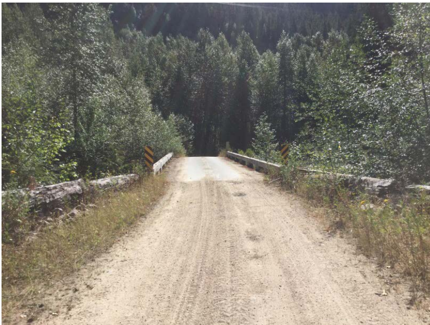
Approach from Right Bank when facing downstream
