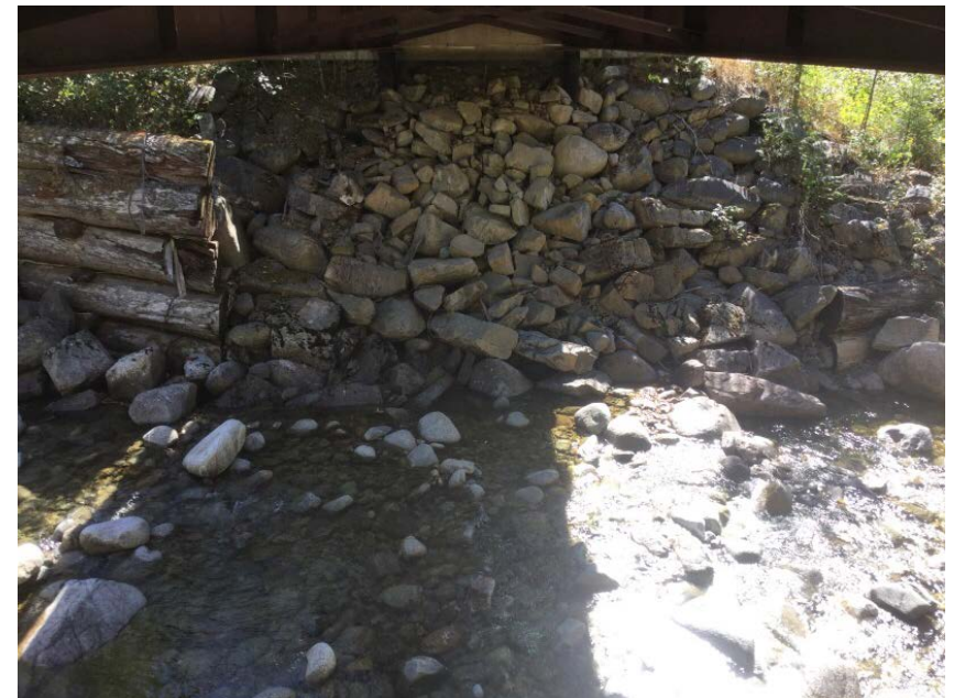
Left Bank Abutment when facing downstream
